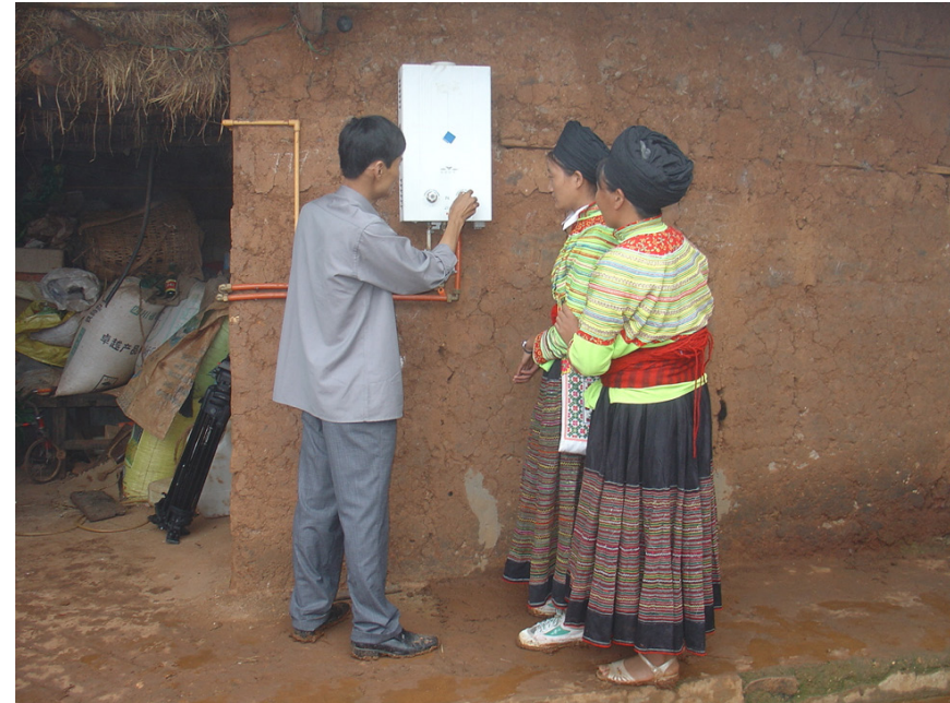
Villagers learn how to use bio-gas as a fuel source for cooking supplied by small-scale anaerobic digesters. Image credit: Sichuan Rural Poor-Household Biogas Development Programme
